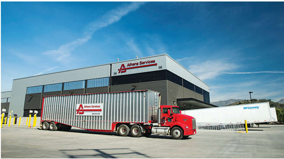
Athens Services Sun Valley Material Recovery Facility
