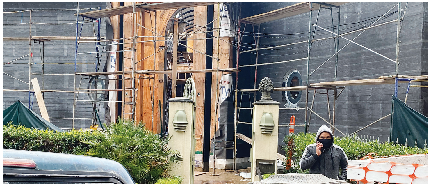
Residential construction continues in the City. Photo by Lisa Bloch
