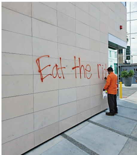
Removing graffiti from the Beverly Hills Chamber of Commerce building
