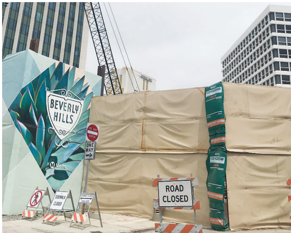
Construction continues on the Wilshire/Rodeo Station. Photo by Laura Coleman
