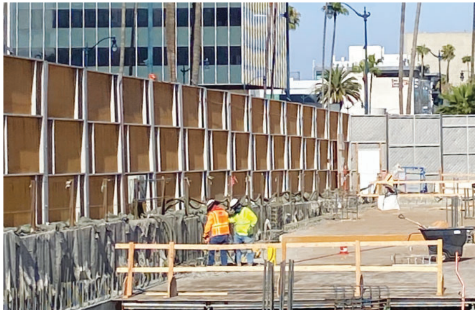
Wilshire/Rodeo station construction
