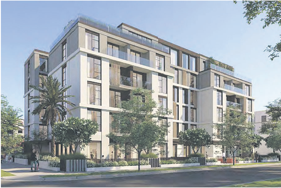
Photo courtesy of Kevin Tsai Architecture
