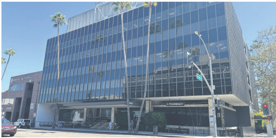
The Wilshire Boulevard site of the planned clinic
