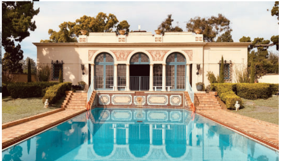
THE POOL PAVILION AT THE VIRGINIA ROBINSON GARDENS UNDER CONSTRUCTION IN 1925 (LEFT) AND TODAY (RIGHT) LEFT PHOTO COURTESY OF THE VIRGINIA ROBINSON GARDENS ARCHIVE; RIGHT PHOTO BY LINDA IMMEDIATO
