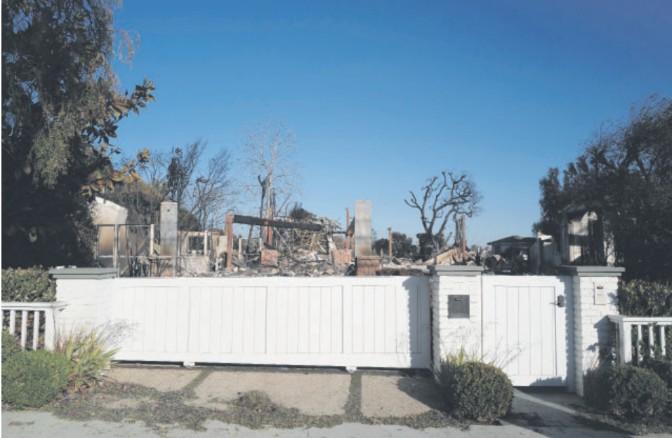
A pristine white gate is all that remains of a destroyed property.
