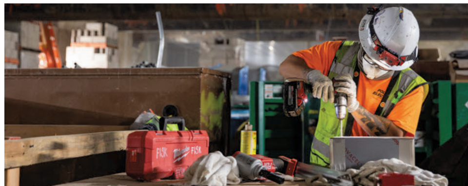
D LINE SUBWAY EXTENSION PROJECT Section 2 – Beverly Hills
