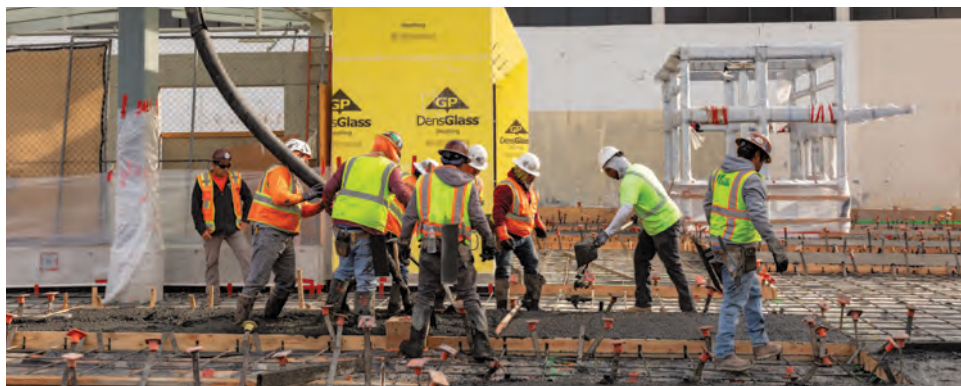
D LINE SUBWAY EXTENSION PROJECT Section 1 – Beverly Hills
