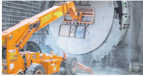
Tunnel Boring Machine in Beverly Hills Photo courtesy of Metro
