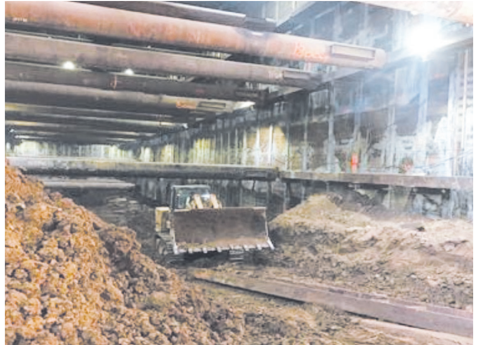
Excavation progress for Wilshire/Rodeo Station box Photo courtesy of Metro
